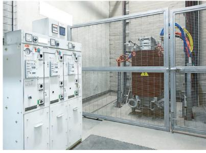
01 Before: The substations were equipped with open medium-voltage cells, following an outdated safety concept.
