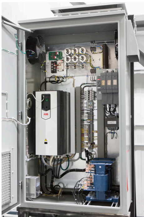
Figure 2. Modern variable speed drives are capable of supporting intelligent artificial lift process control and protecting the equipment through remote monitoring.
