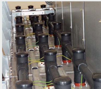
Busbar compartment with support for voltage transformers
