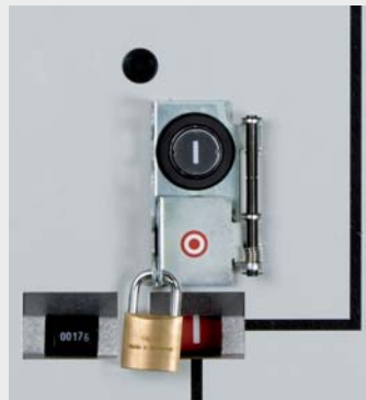
Secured to prevent deearthing
