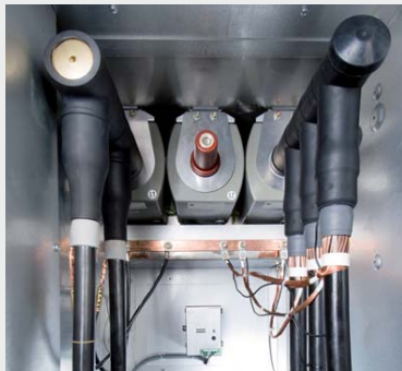
Cable compartment with current transformers
