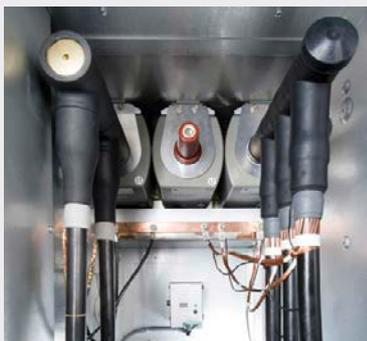
Cable compartment with current transformers
