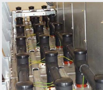
Busbar compartment with support for voltage transformers
