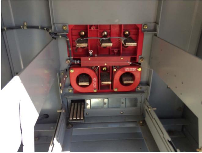
Fig. 8 Trigger wire on line side stabs in feeder breaker compartment.
