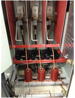
Fig. 14 An example of a 3 pole HSGS retrofit
