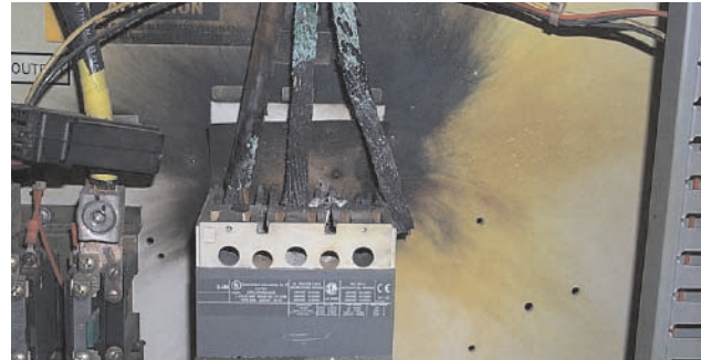
Photo 3, Arcing Caused by Loose Input Contacts
