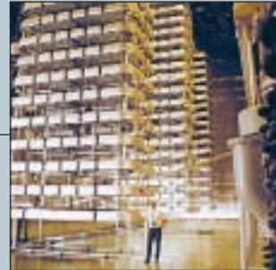
**Mercury-arc valve based HVDC had come a long way in a short time, but it was a technology that still harbored some weaknesses. One was the difficulty in predicting the behavior of the valves themselves. As they could not always absorb the reverse voltage, arc-backs occurred. Also, mercury-arc valves require regular maintenance, during which absolute cleanliness is critical. A valve that avoided these drawbacks was needed.**
