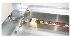
Figure 73: connection to the busbar in an MV panel
