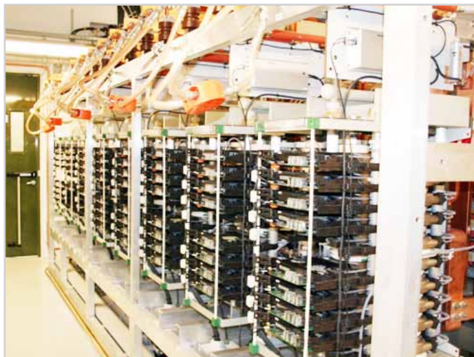
One of the two converters PCS 6000 with earthing connections. Each converter is capable of delivering 15 MW to the railway grid
