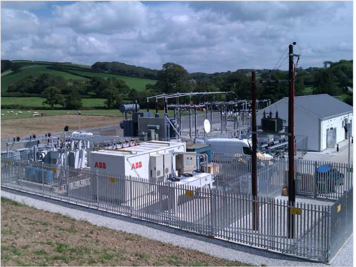
Overview of the STATCOM installation in Fullabrook Wind Farm, UK
