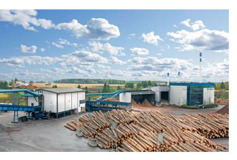
At the Westas sawmill in southern Finland, the long production process is all about conveyor technology. Different pieces are transported; in the beginning of the process, they are heavy logs and then as different smaller pieces. For the process to flow smoothly, the conveyors use variable speed drives for flexible and accurate speed control.
