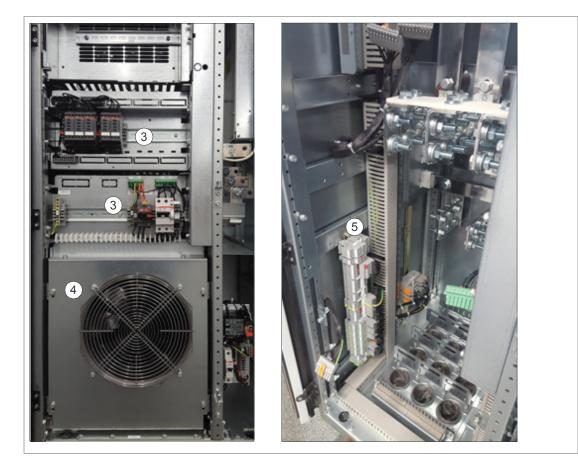
6. <u>Bottom entry:</u> Route the cables to the control unit (a), additional terminal block X504 (option +L504) as shown below.
