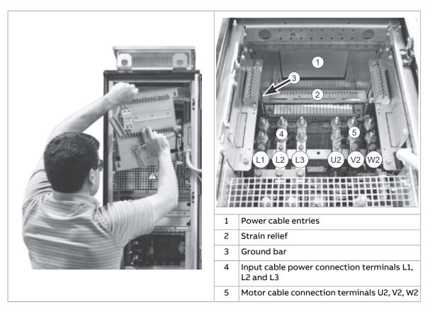
This figure shows the layout of the power cable connection terminals of frame R11.
