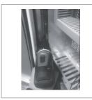
**Note:** You can access the screws on the left side of the fuse shroud easier if you open the swing-out frame slightly and use the gap between the swing-out frame and cabinet frame to access the screws.
