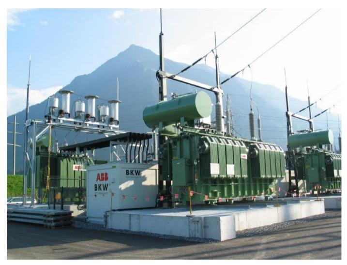
ABB 20-MW-Converter – 4 Units 3AC 50 kV 50 Hz – 2AC 132 kV 16,7 Hz 84 MVA / 80 MW
