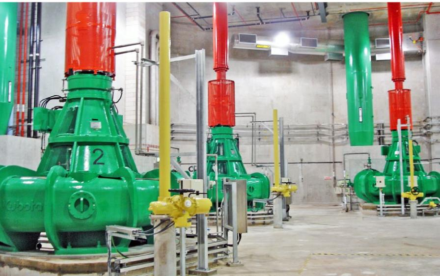
— Pumps in one of the two giant pump shafts at the Changi influent pumping station. The pumps are controlled by ABB's ACS1000 drives.
