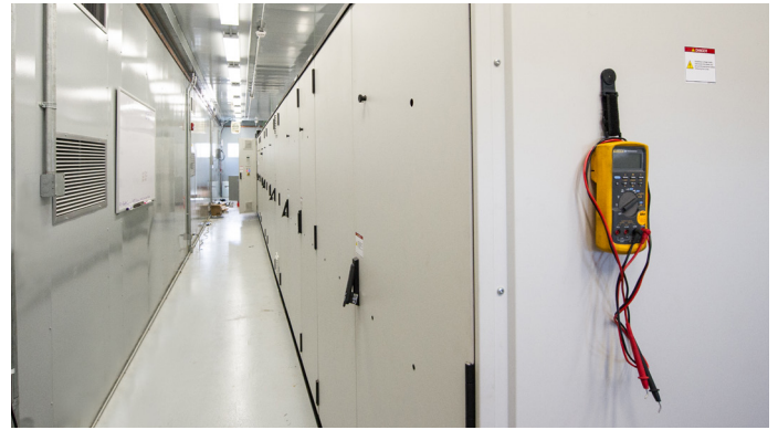
The ACS6000 Controllable Grid Interface (CGI) has considerably reduced the time and cost of certification of wind generators. (Photos of the inside of the CGI. Photo by Dennis Schroeder/NREL)
