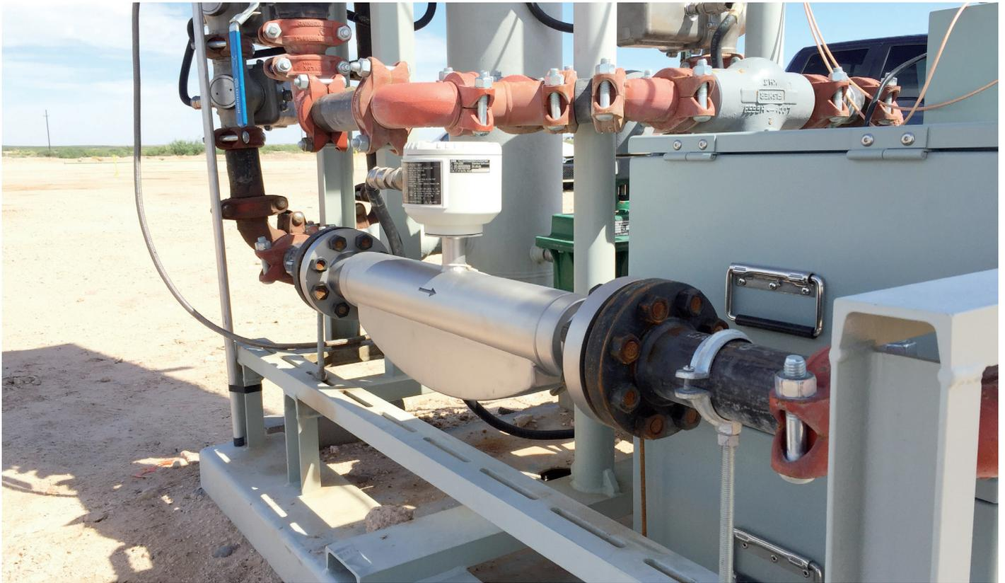
CoriolisMaster in upstream O&G – installed with ABB's Field Information Manager.
