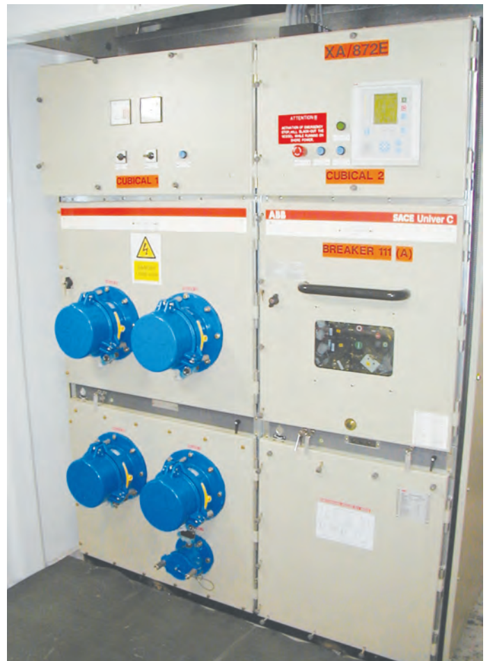
Figure 2 shows a ship with diesel machinery and low voltage electric system. The shore-to-ship power system is arranged with the shore connection panel located outside the main switchboard room with cable connectors mounted in the front. An onboard transformer steps down the power from high to low voltage.
