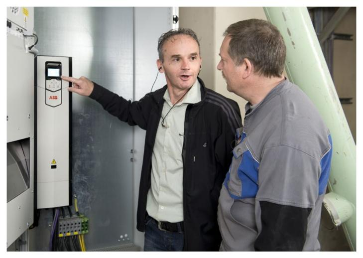
Sensors are used in the ventilation system for measuring the temperature and humidity of the exhaust air. The operator can respond, if necessary, to the changing air values with the frequency converter and optimize the air flow rate.
