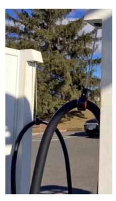
ABB offers a field-mounted cable management solution that keeps charging cables off the ground whether in use or when the connector is stored.
