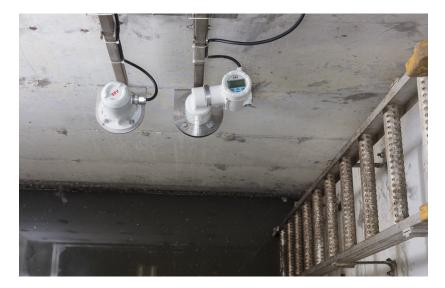
LLT100 detects clear liquids, allowing new applications for laser level measurement.
