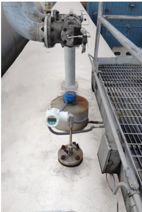
LMT100 insertion type magnetostrictive liquid level transmitter
