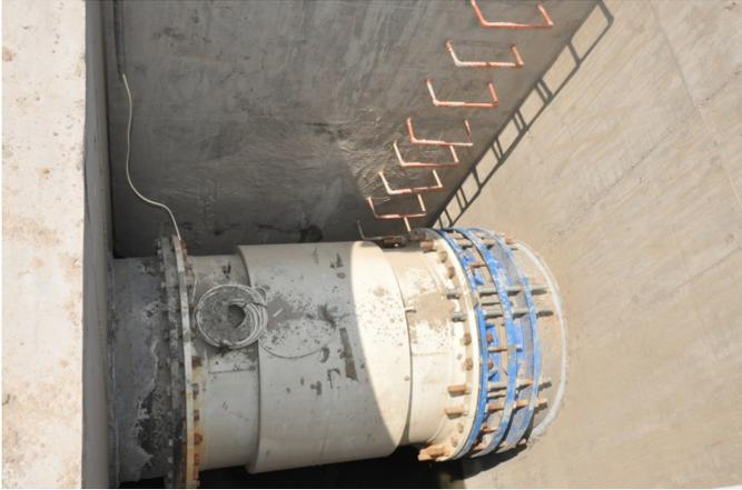
**ABB WaterMaster magnetic flow meter prior to being submerged in pit**
